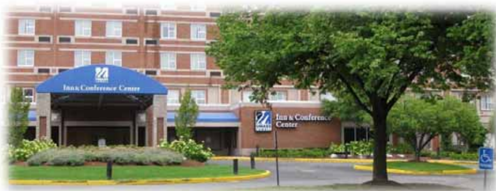
Inn & Conference Center 50 Warren Street, Lowell, MA
